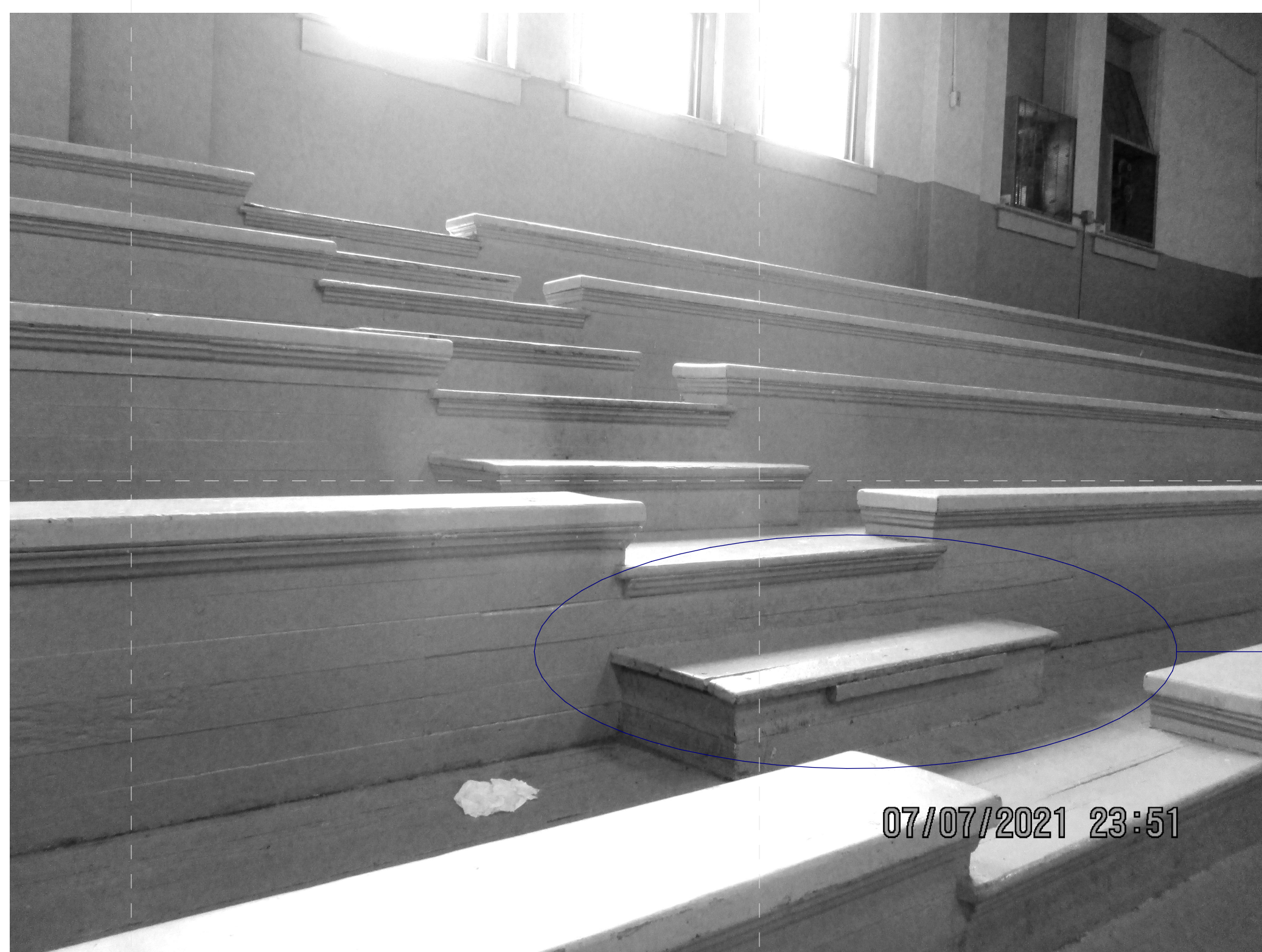
Example of Typical Repair
