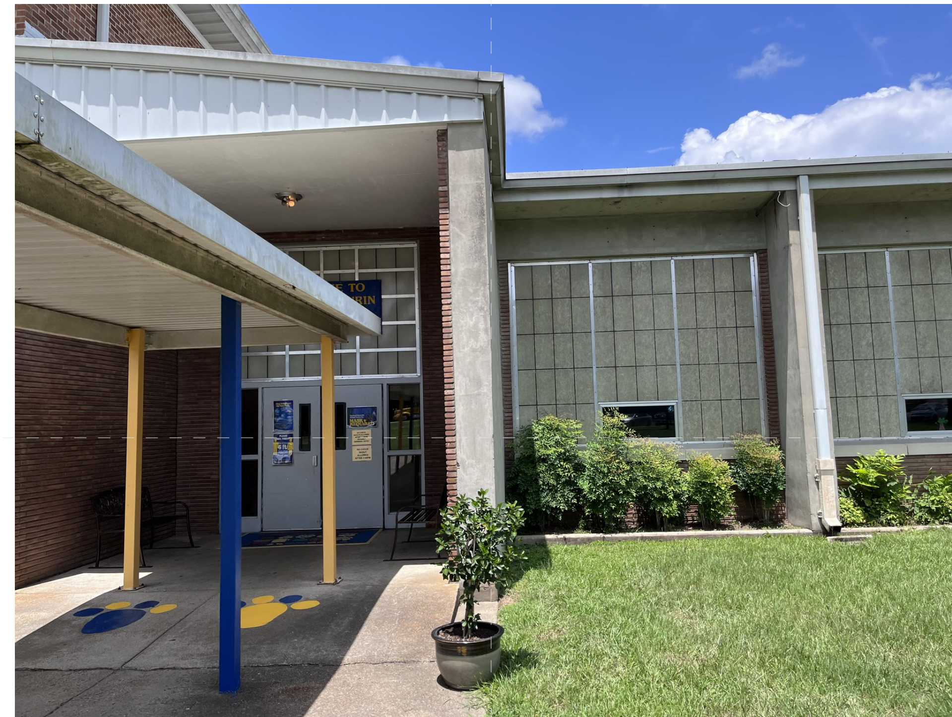
Entry Double Doors to be Replaced
