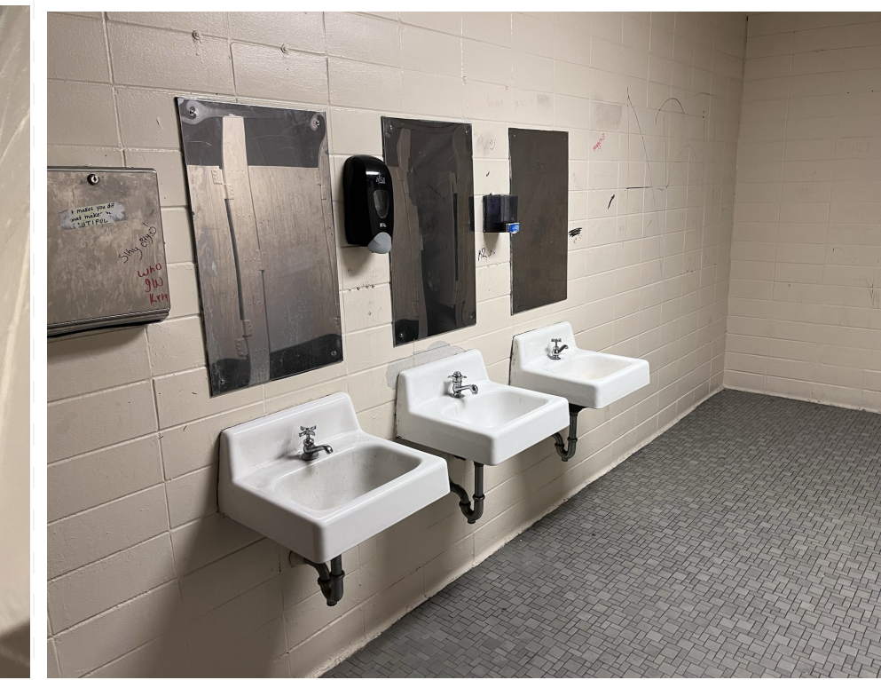
Typical Toilet Lav Wall
