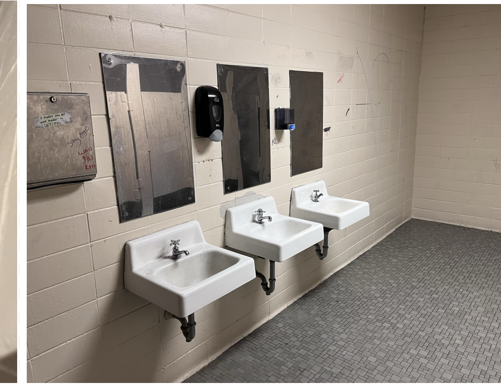
Typical Toilet Lav Wall
