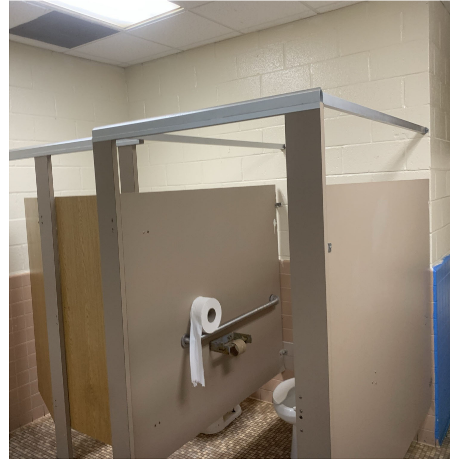
Typical Toilet Room
