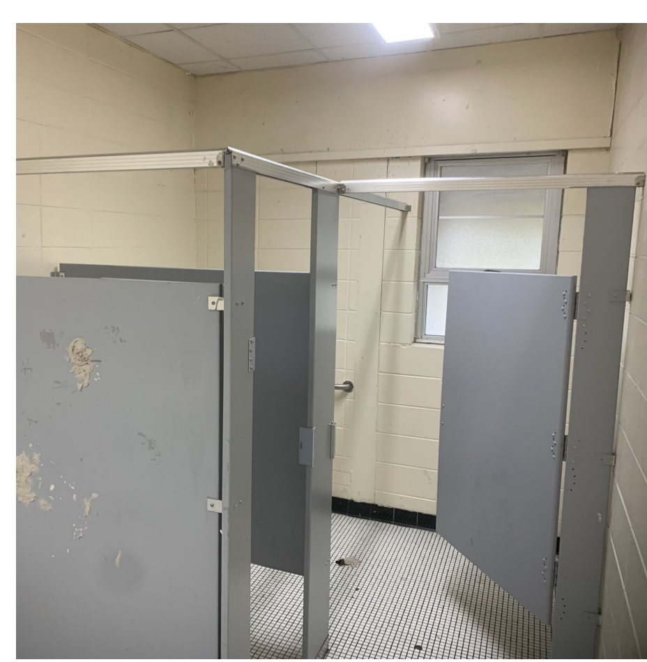
Typical Toilet Room
