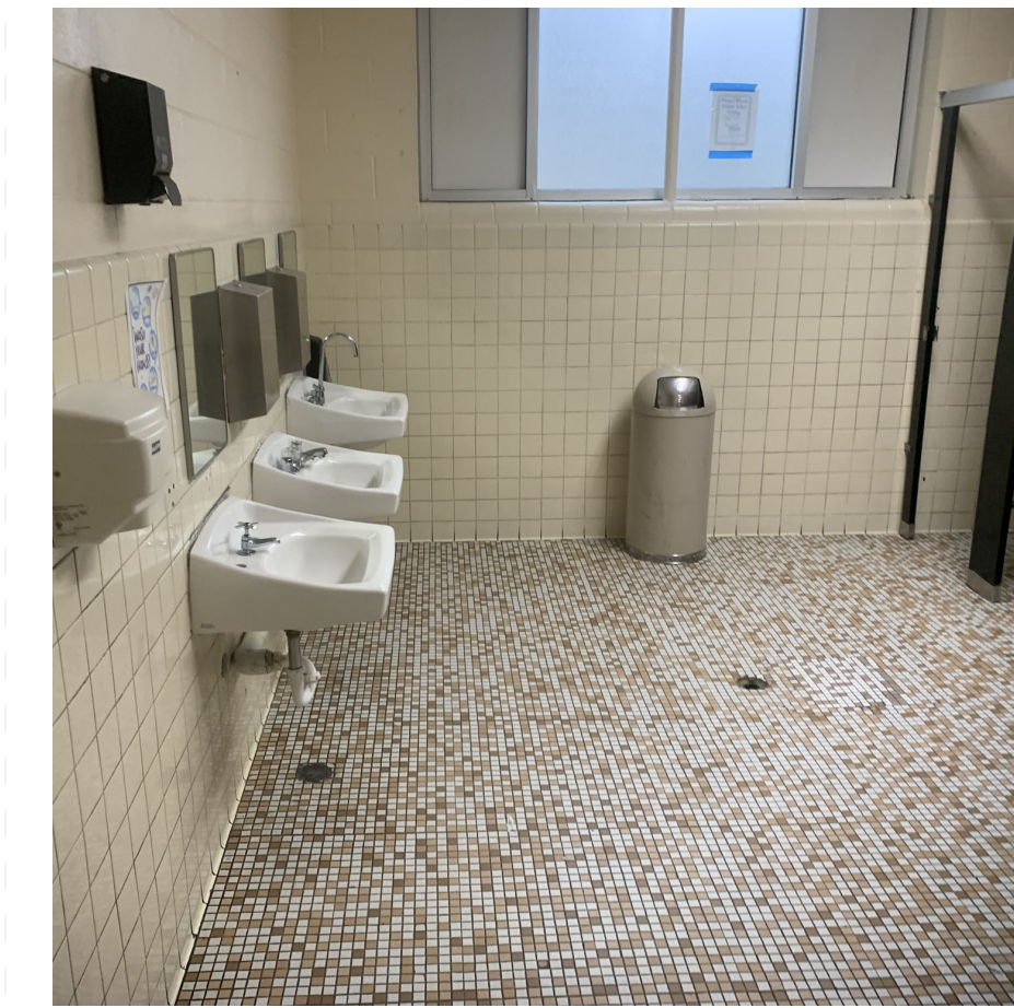
Typical Toilet Room
