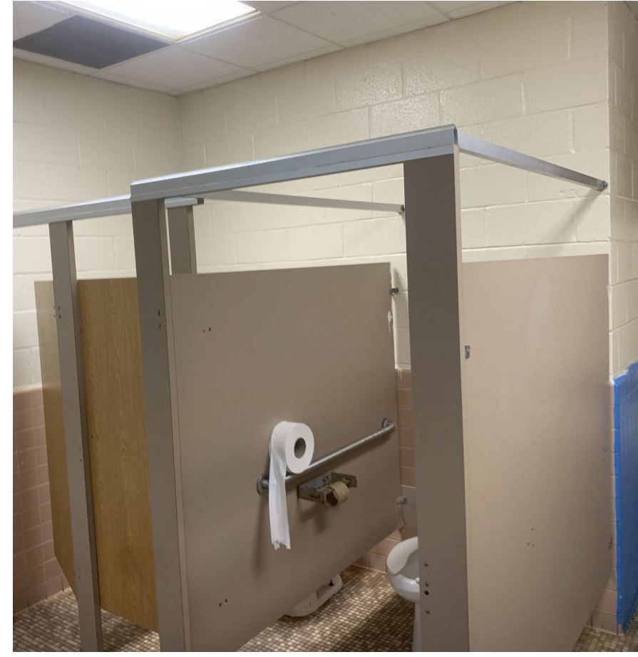
Typical Toilet Room
