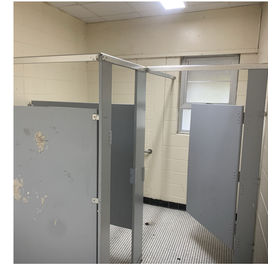
Typical Toilet Room
