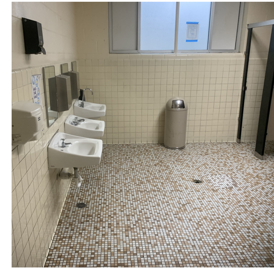
Typical Toilet Room
