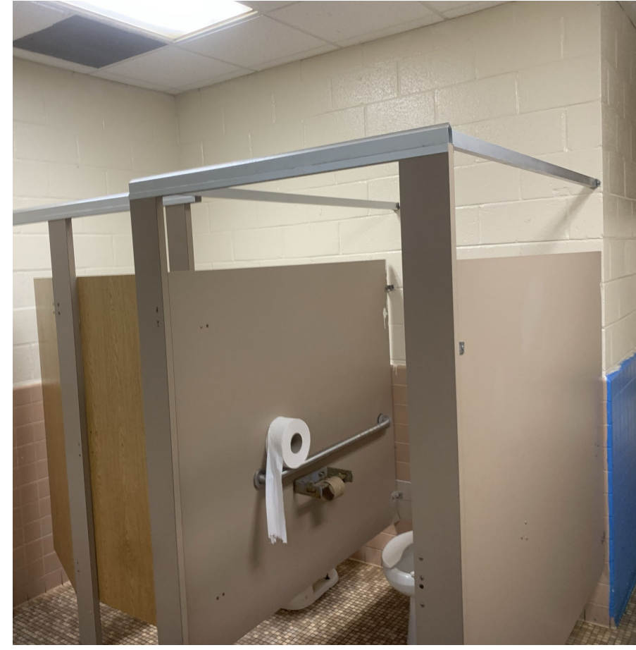
Typical Toilet Room
