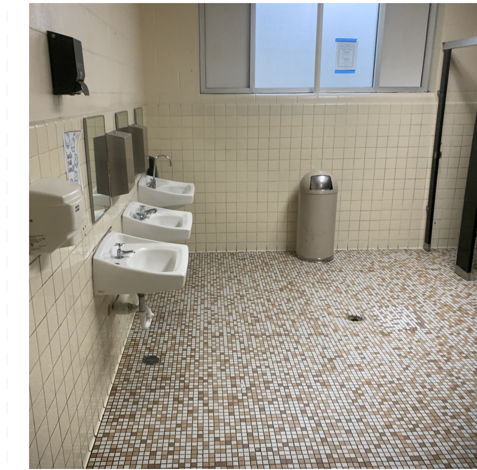
Typical Toilet Room
