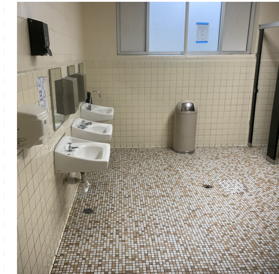
Typical Toilet Room
