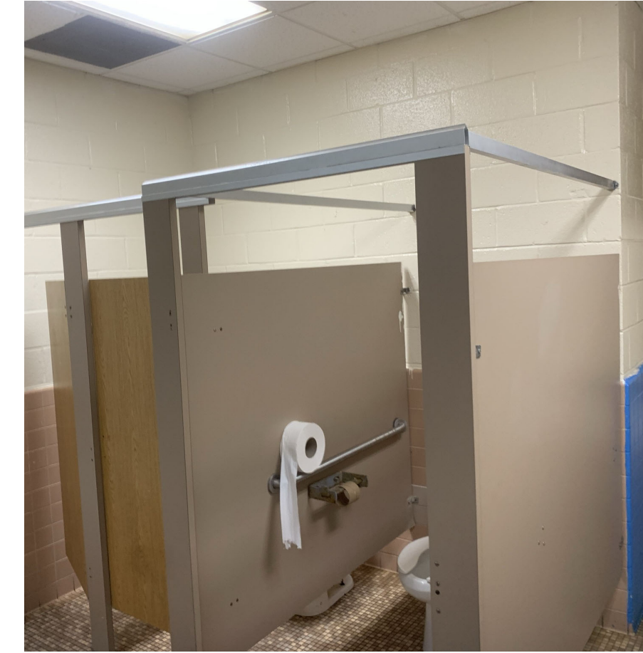
Typical Toilet Room
